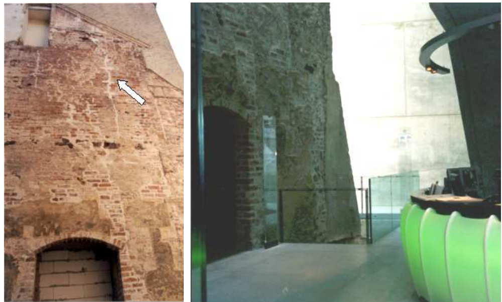
Figure 1. Luther House Wittenberg, Germany, Westem gable: situation before and after erecting the new entrance building. The complete gable was investigated with radar in order to detect hidden voids and other irregularities.
