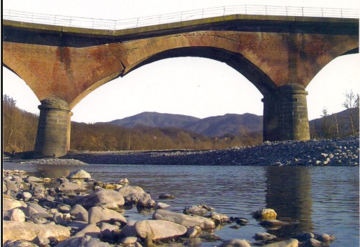
Road bridge Arquata S., Alessandria
