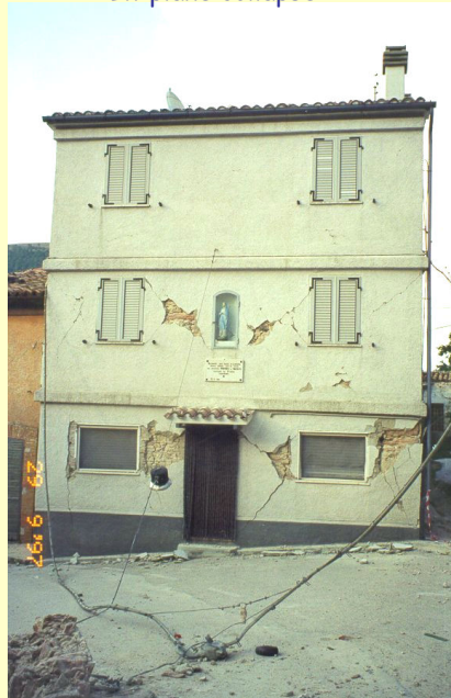
In-plane collapse
