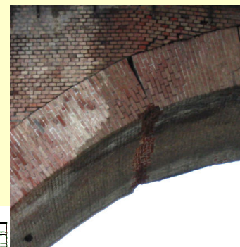
Generalized hinge at a masonry arch
