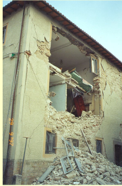
Out-of-plane collapse
