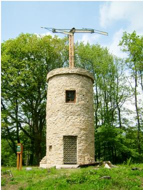
“Le système Chappe: The world’s first (wireless) telegraph network developed by Napoleon, carrying digitally-encoded text messages across 19h-Century France via optical signals relayed by a network of repeating stations extended from Lyon to Venice”
