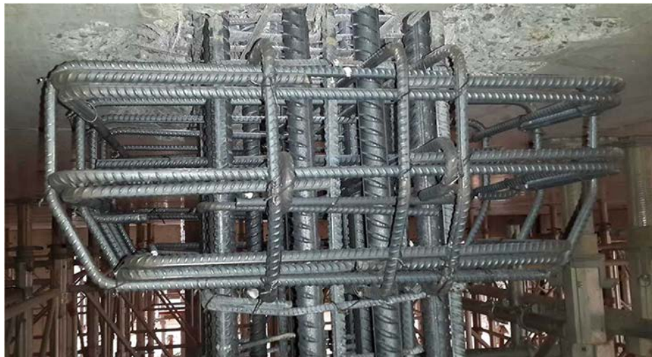
Corbel reinforcement
