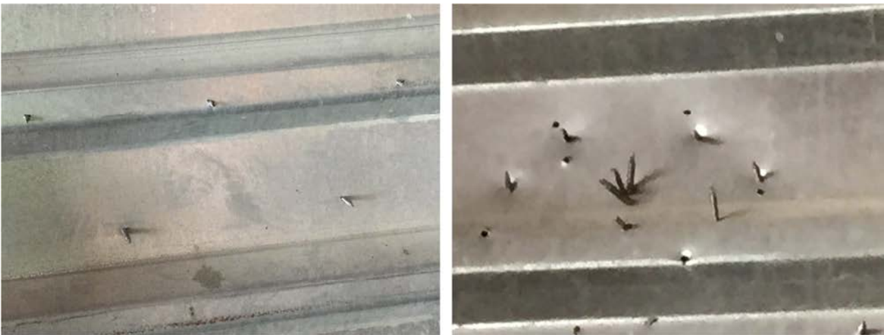
Pedestal to metal decking connection
